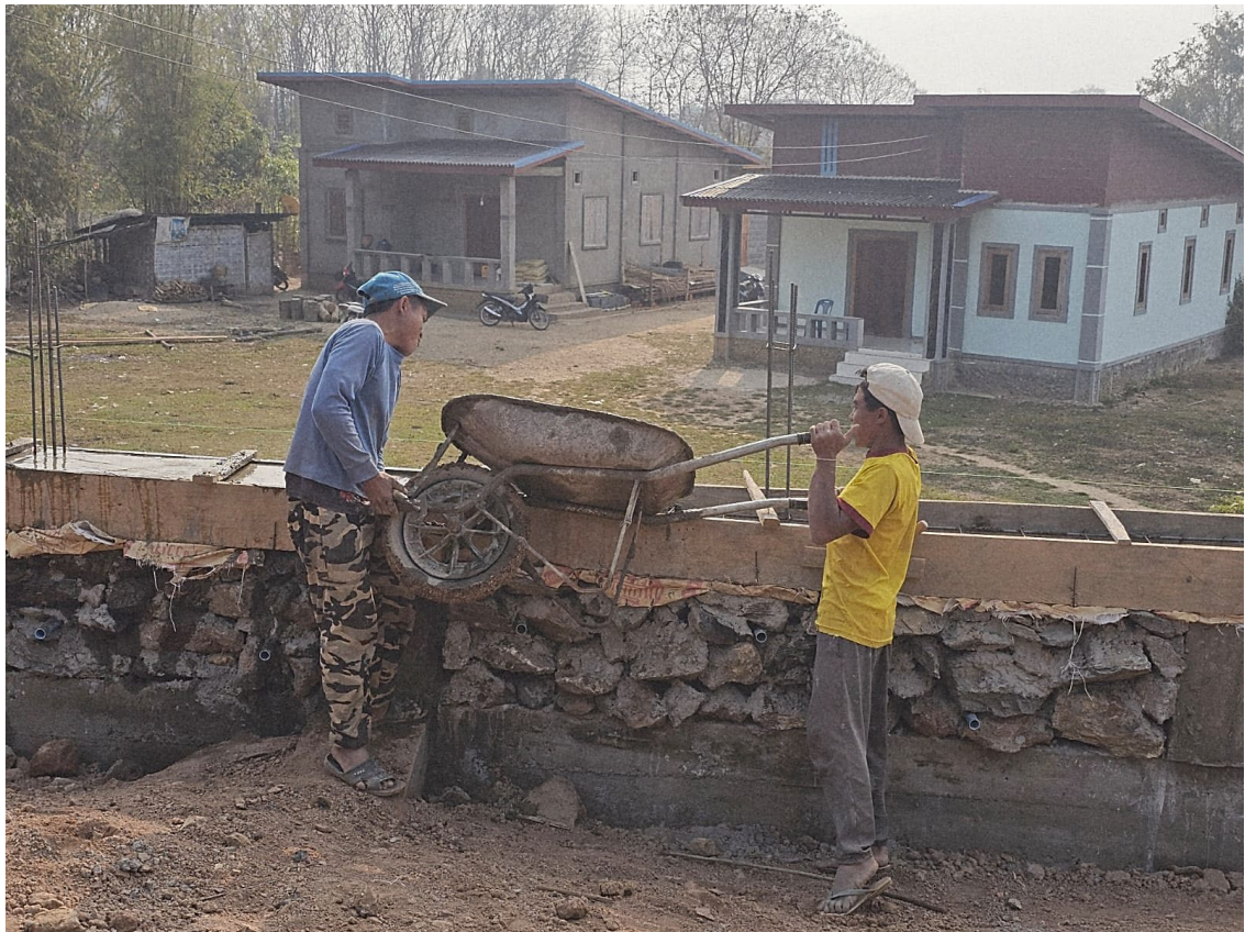
Rebuilding Failed Retaining Walls in Houn
