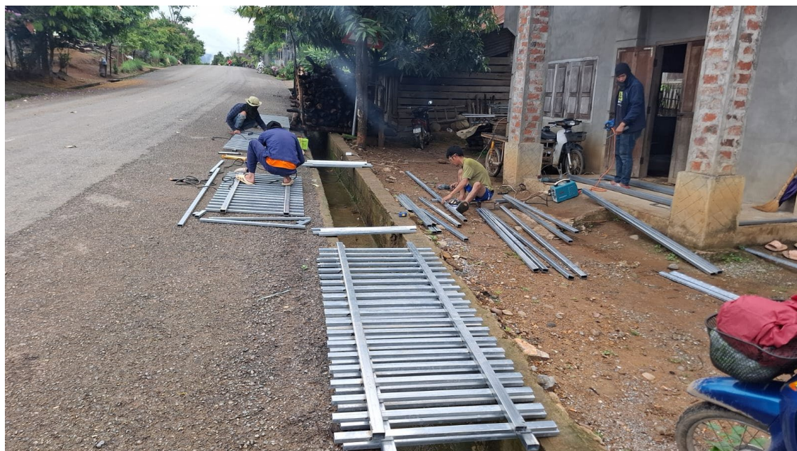
Construction of a Fence for Houn Eye Care Clinic Building Site
